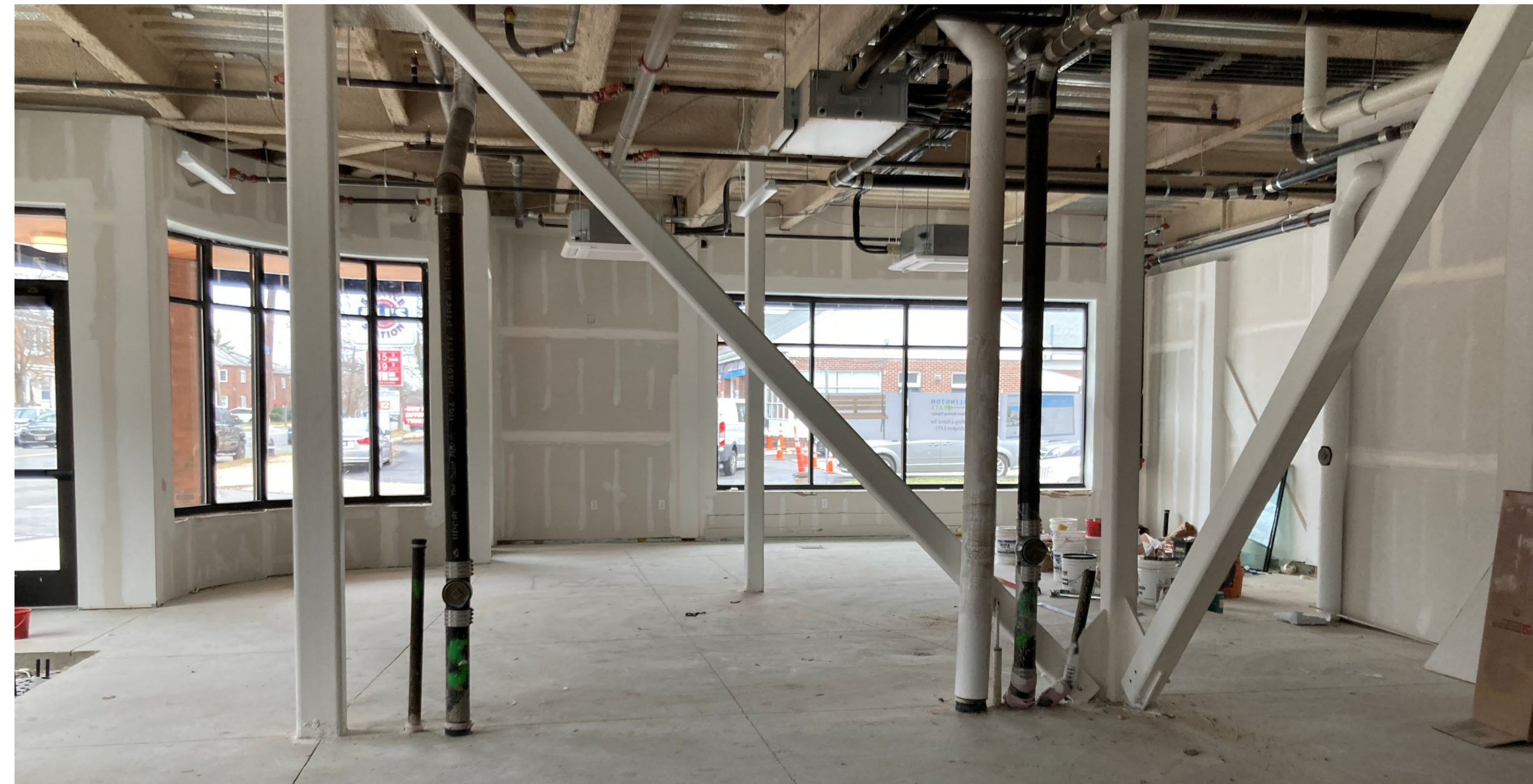
Construction Process – Existing Conditions - Arlington EATS
